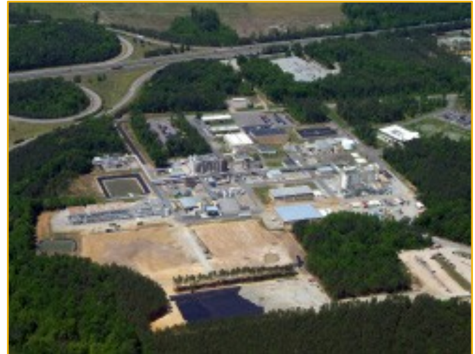
Production areas at Boehringer Ingelheim Chemicals plant in Petersburg, VA, are deemed hazardous, requiring an intrinsically safe fieldbus installation.
