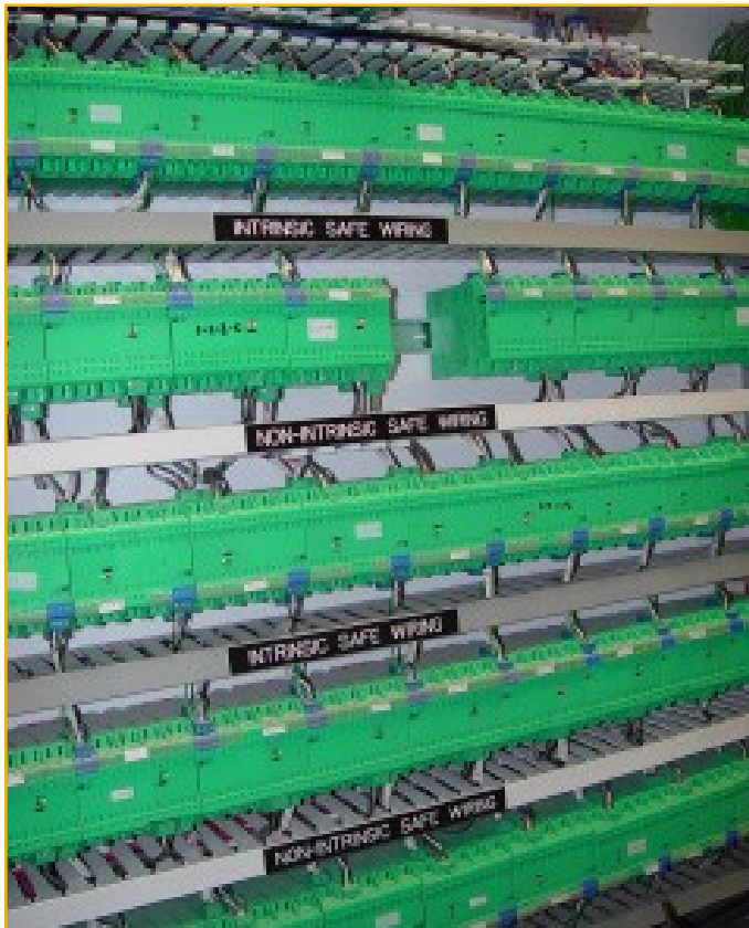
Figure 4. The original ENTITY-based IS system, installed in 2001, required barriers, large cabinets and many fieldbus segments.
